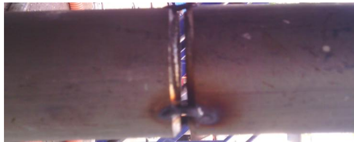
Figure 2. Tack welding at both 304 stainless steel pipe
