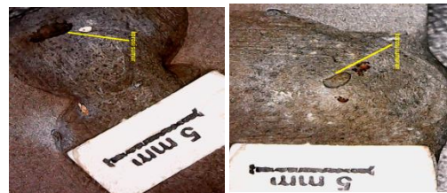
Gambar 4. korosi sumur ( pitting corrosion )
