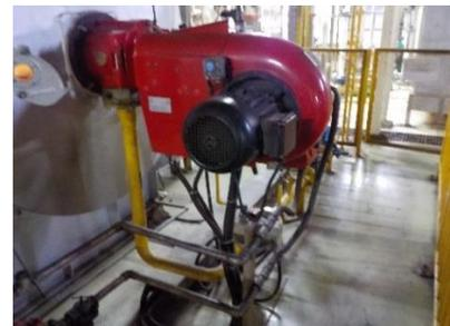
Gambar 2. *Burner Weishaupt tipe RGL dual fuel burner*
