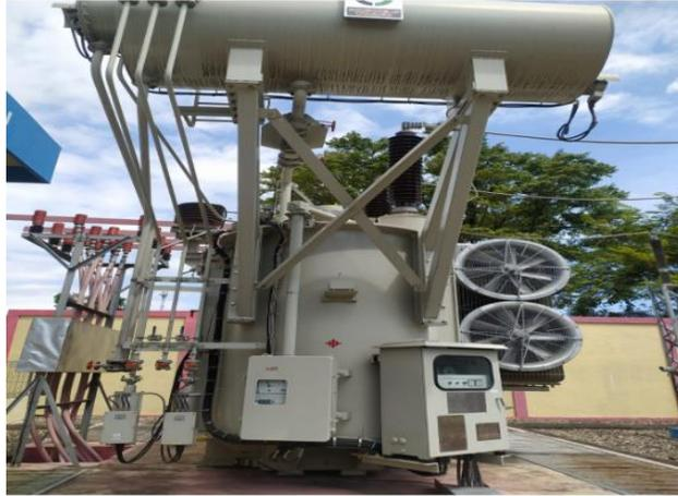
Gambar 1. Transformator Daya III GIS Simpang Haru(Gupta dkk., 2000)
